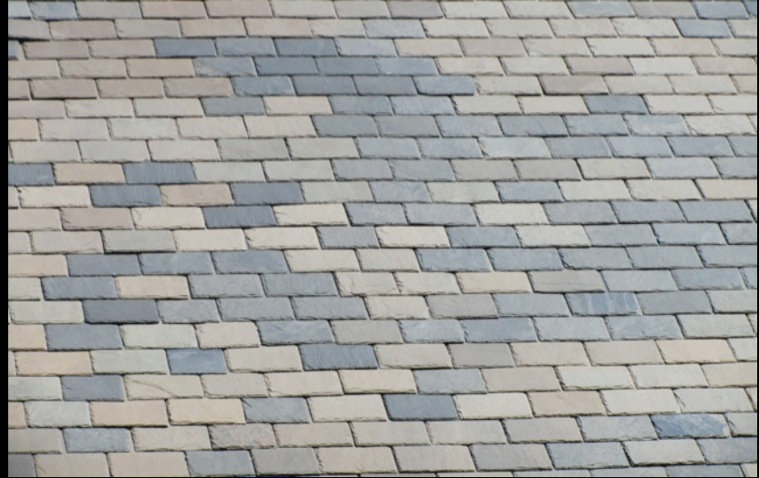
Uniform width slate roof
