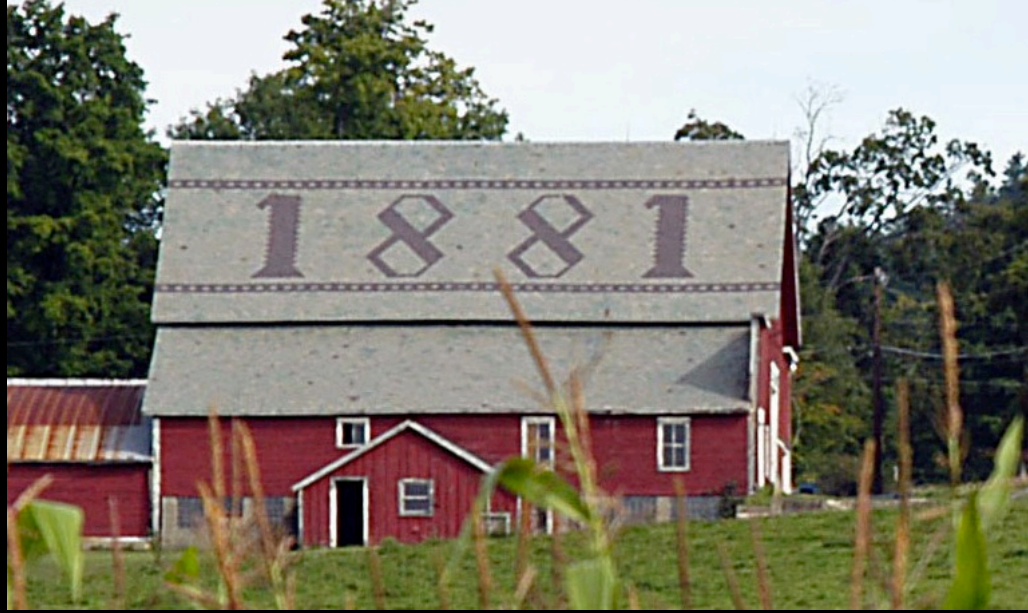
An S-1 slate roof has at least a 75-year lifespan. Photo courtesy of Hathaway Farm, Rutland, Vermont
